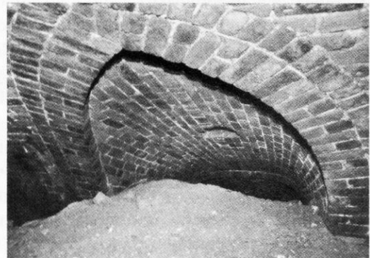
Gothic arch in the backfilled third level below Paddington Photo by Chris Iles
